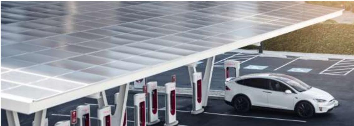
Figure 11. Off-grid charging station developed by Tesla [63]
